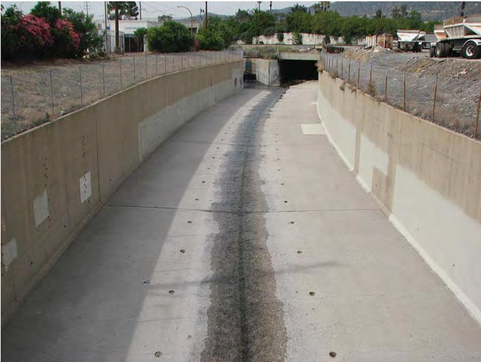
PHOTOGRAPH 2. Concrete-lined rectangular open channel upstream of Discharge Point 002 looking upstream toward the northwest.
