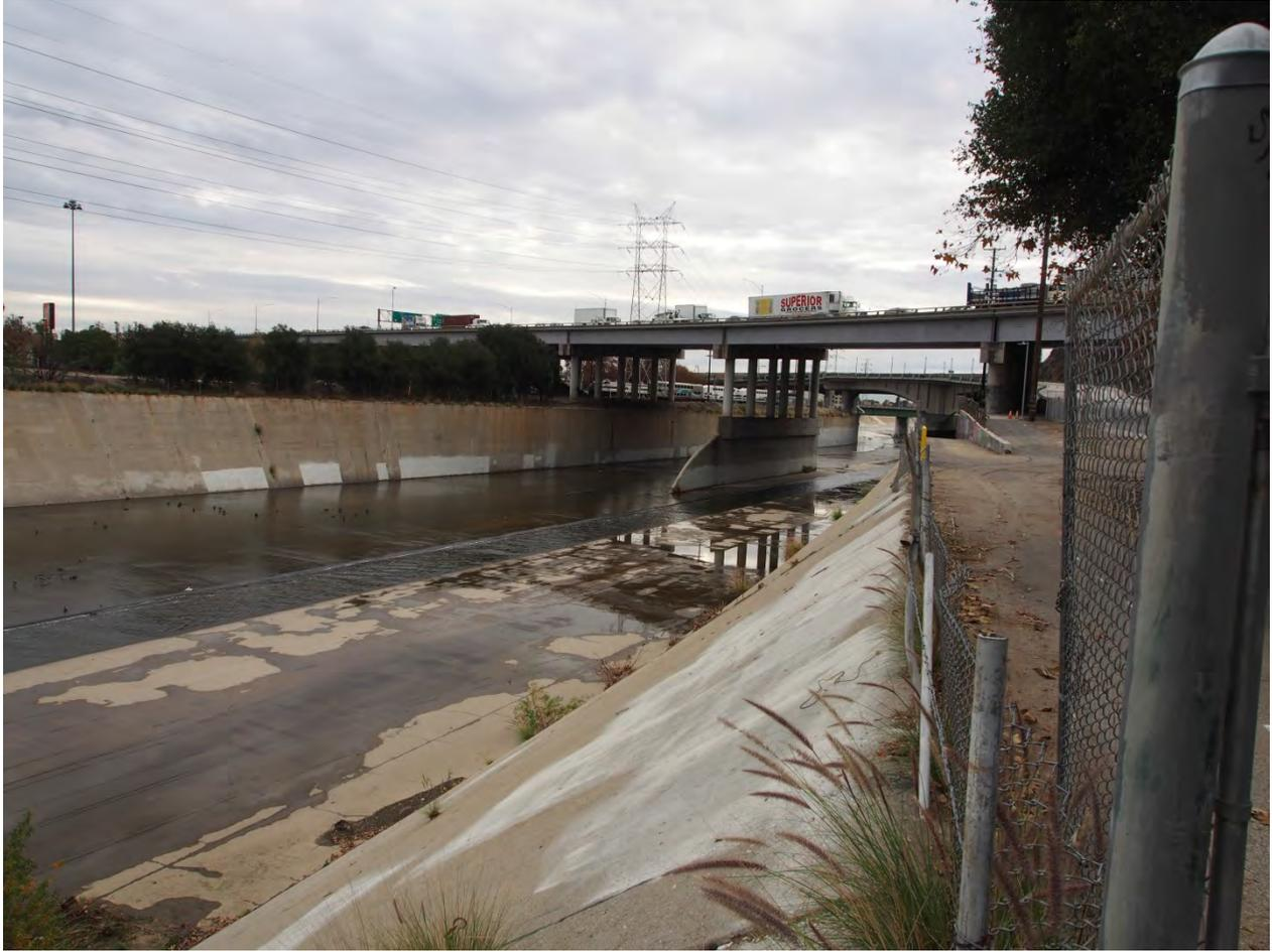
**Photo 20:** Depicts the transition at the southern end of Segment 5 to concrete bottom of Segment 6, where the River forma a thin sheet of water at the edges of a deeper, fast moving center channel. Photo was taken from the bike path facing southeast.
