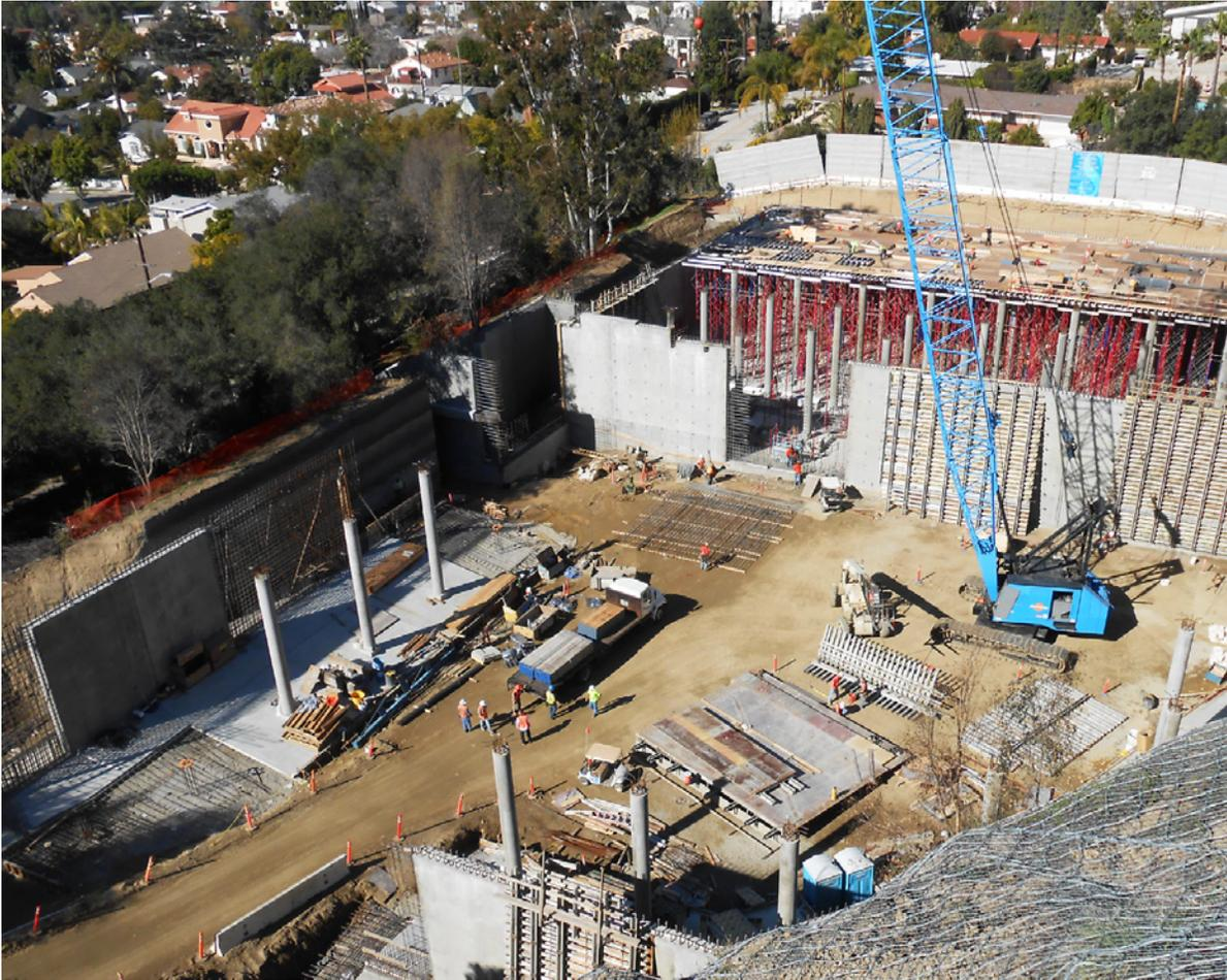
The reconstruction of Reservoir 1 replaced a vintage 1928 obsolete and leaky reservoir near the intersection of Sunset Canyon and Magnolia Boulevard with two reservoirs with a combined 40% greater storage capacity. The new reservoirs are constructed to modern day seismic and structural standards, are less visible, fit into the same physical area, and have a zero leak rate.
