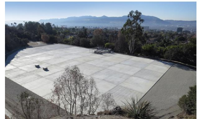
The reconstruction of the Reservoir 1 increased the water storage capacity from 6.9 million gallons of water to 9.5 million gallons.
